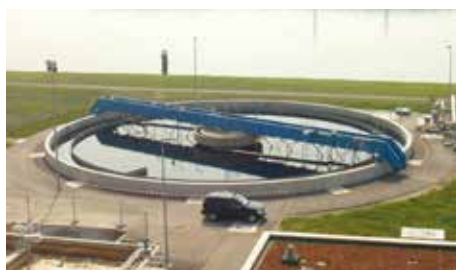
▪ HIK Doppel-Rundschildräumer / HIK double circular-tank shield scraper
